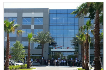
The Verizon Lake Mary Finance Center Building
